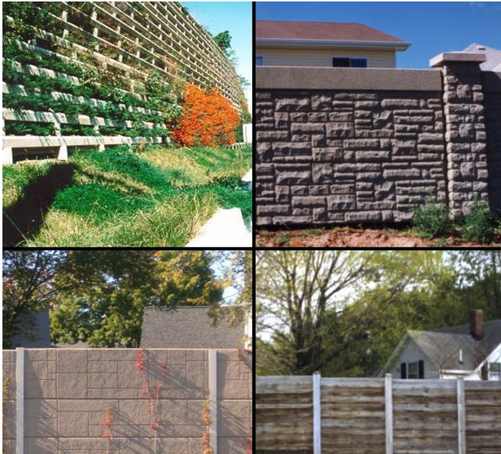
Figure ES-8 Examples of Noise Barrier Materials
